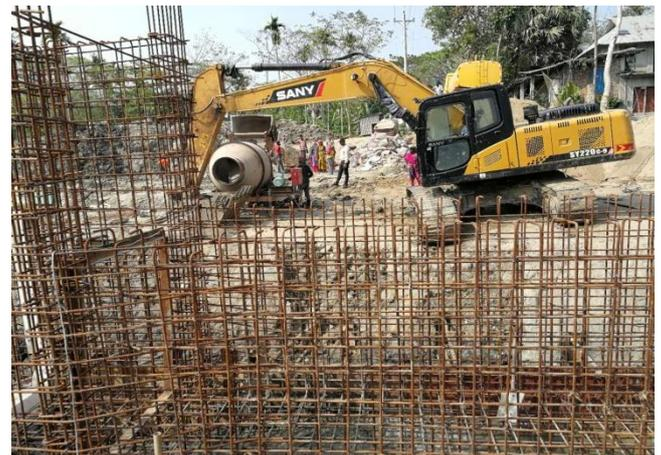
Figure 3-65: Pouring the RCC Box Base Slab For DS-9 of Polder-41
