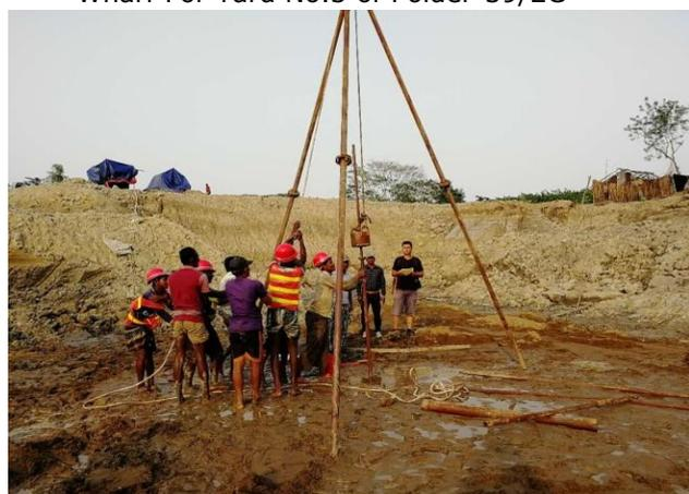
Figure 3-61: Drilling the Dewatering Bore Hole For DS-5 of Polder-40/2
