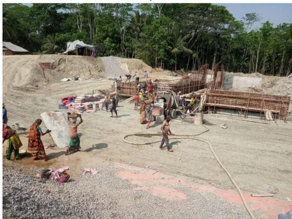
Figure 3-66: Pouring the RCC Wall for FS-1 of Polder-41/1
