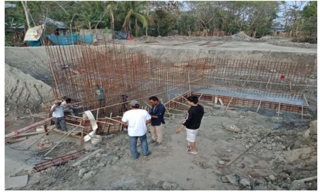
Figure 3-63: Fixing the Deformed Bar For FS-10 of Polder-40/2
