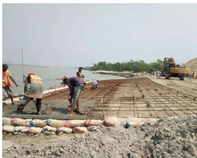
Figure 3-59: Pouring The Concrete For The Wharf For Yard No.3 of Polder-39/2C
