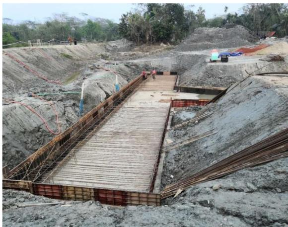
Figure 3-68: Establishing the LC form for DS-7 of Polder-43/2C
