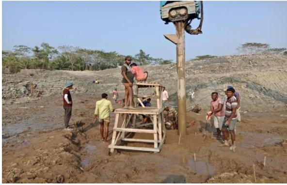
Figure 3-62: Executing the Sand Pile For DS-5 of Polder-40/2
