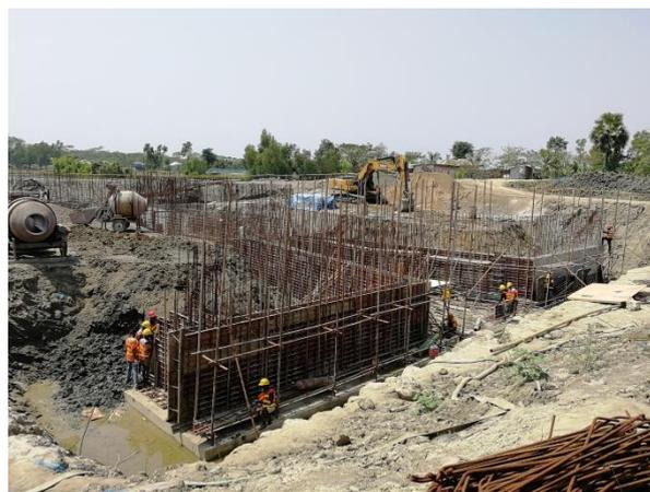
Figure 3-69: Establishing the Form for RCC Wall for DS-3 of Polder-47/2
